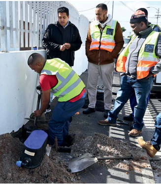
Getting stuck in: Mayoral Committee member for Water and Sanitation Cllr Zahid Badroodien (in the black jacket) with a team on-site in Athlone carrying out a water meter replacement.
